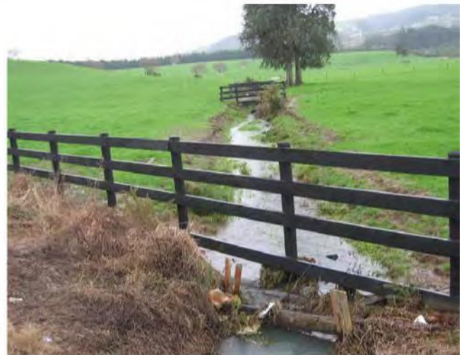
LOCATION E (FIG 2) - The northern stream at the base of the northern escarpment will be rehabilitated as part of the proposed works
